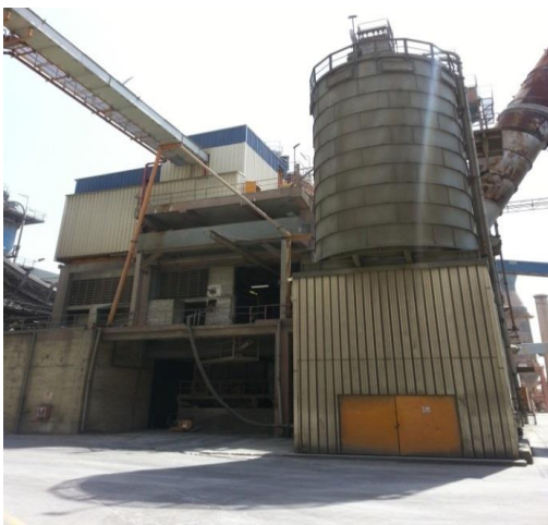
Figure 3. Silo of combustible fuel of line 7.
